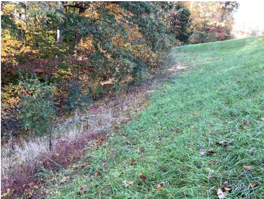
Top: Downstream slope at left abutment; note trees and brush within 25 feet
